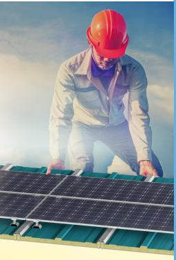
Thanks to its special clamp system, Solar Capped Panel is easily mounted on the surface of Assan Sandwich Panel without drilling any screw holes. As it is installed without drilling on the roof, it offers excellent waterproofing performance and high corrosion resistance as well as extending the economic life of the buildings by maintaining the structural integrity of the roofs. In addition, it offers cost efficiency in steel construction with its design allowing for low slope
